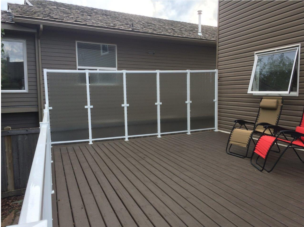
Figure 1 6-foot Wind Wall
