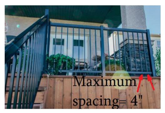
2. Openings through any guard that is required by Article 9.8.8.1. and that is installed in a building of industrial occupancy shall be of a size that will prevent the passage of a spherical object having a diameter of 200 mm unless it can be shown that the location
