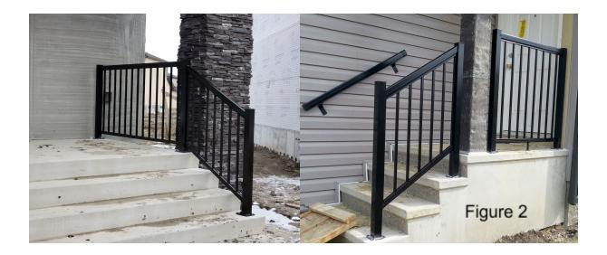
**Figure 1:** The railing extends from the bottom step to the landing, indicating a pass of code **Figure 2:** The grab rail extends from the bottom step to the landing, so even though the railing on the right does not extend all the way to the landing, it will still pass code because it is just acting as a guard.
